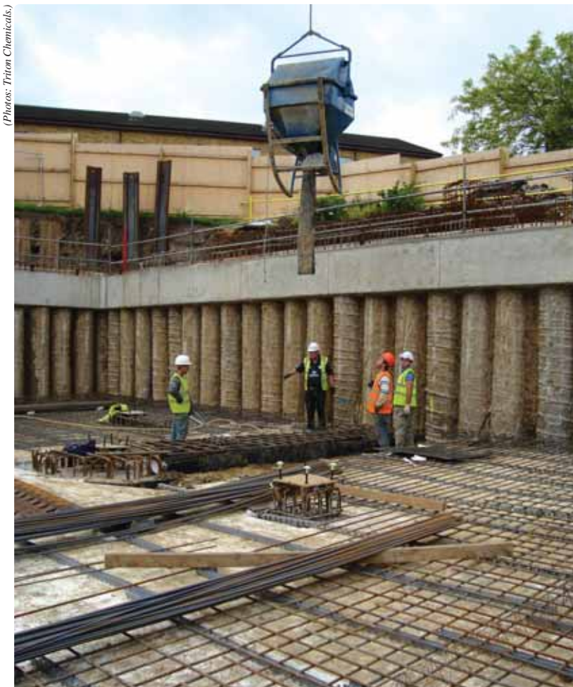
Figure 1: Basement construction in progress at Goldsmiths, UCL.
